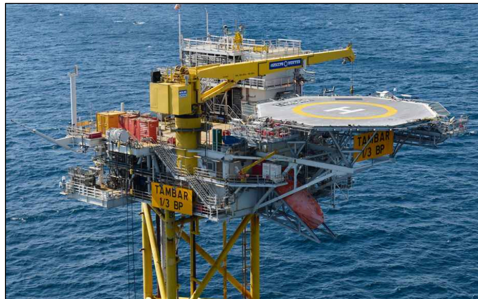
Normally Unmanned Installation (NUI) - Norway
